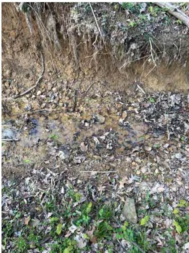
ID: S-BS-5-1 Date: 4/14/2026 Direction: S Position: Across
